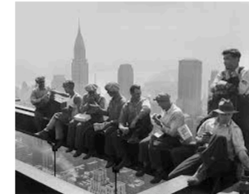
1932 Photo Of Workers On A Steel ... businessinsider.com
